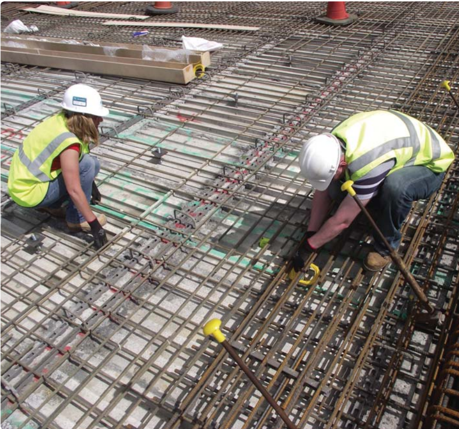
Figure 5: Positioning of BFRP bar with fibre bragg grating sensors.
