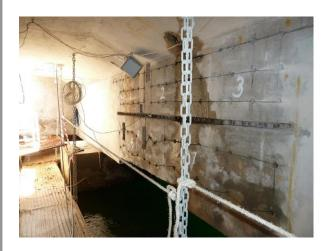
As part of the renovation works the client requested a corrosion protection system to protect the worst areas from further corrosion related deterioration. 5000 DuoGuard Hybrid anodes were installed on the underside of the deck, on the front and rear faces of the service duct and headstocks.
