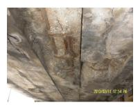
The corrosion protection system was designed to ensure an extended 25 years of jetty service. The DuoGuard Hybrid System consists of an initial impressed current phase which passivates the corroding reinforcing steel within the structure. The system is then put into the second, galvanic phase to maintain the steel in a passive environment.
