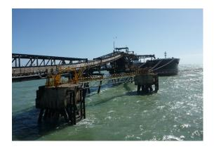
Over 8000 DuoGuard Hybrid anodes were installed to the Kentledge Beams of Bays 1-7 and 12-18. To allow for continuous monitoring of the system, MN15 reference electrodes were installed at 5 representative locations, with the facility to determine steel corrosion rates as requested by the client.
