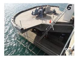
The DuoGuard Hybrid corrosion protection system was determined to be the most suitable solution to prevent further corrosion damage to the dolphins. The DuoGuard anodes were installed in four zones on each dolphin. The anodes were installed on the soffit and the lower 200 mm of the side walls to protect the concrete areas subject to high tide immersion and splash.
