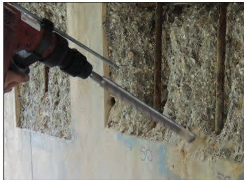
1. Drill the hole into the parent concrete.
