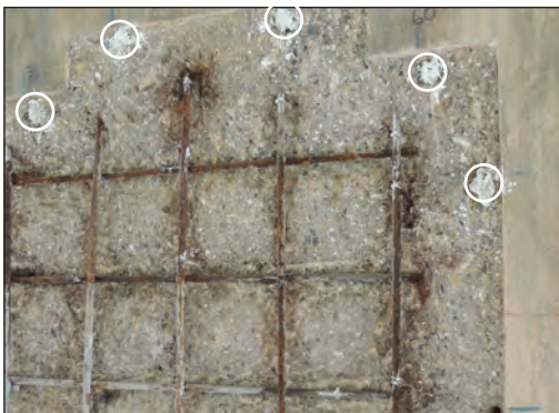
5. Completed PatchGuard installation prior to repair mortar application.
