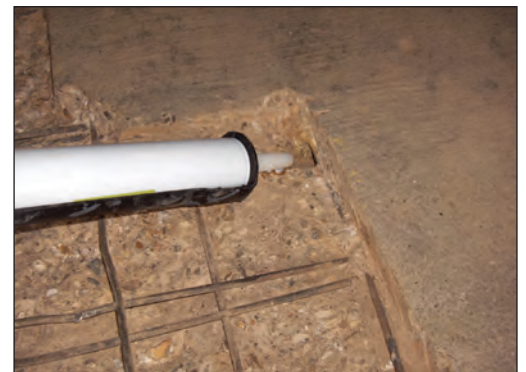
2. Apply the embedding mortar (DuoCrete PG).
