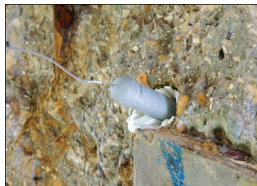
3. Simply insert the anode into the embedding mortar.
